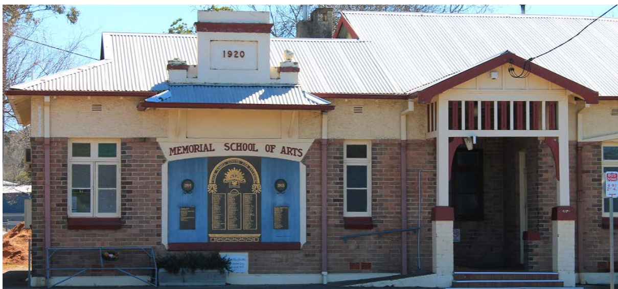
School of Arts building, Coolah
